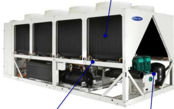
Inverter-driven Carrier screw compressor & reliable air-cooled VFD (30KAV-ZE)
