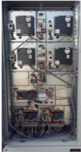
Fan drives + Pump drives + electronic boards
