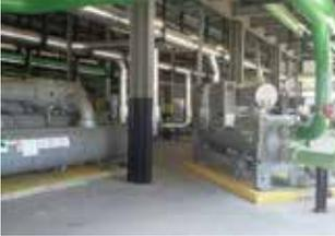
*Even though we have not fully completed automation of the chilled water system, the Carrier 23XRV chillers are operating very close to factory performance, which we consider highly satisfactory. We anticipate seeing an even better coefficient of performance once automation is complete.”*
